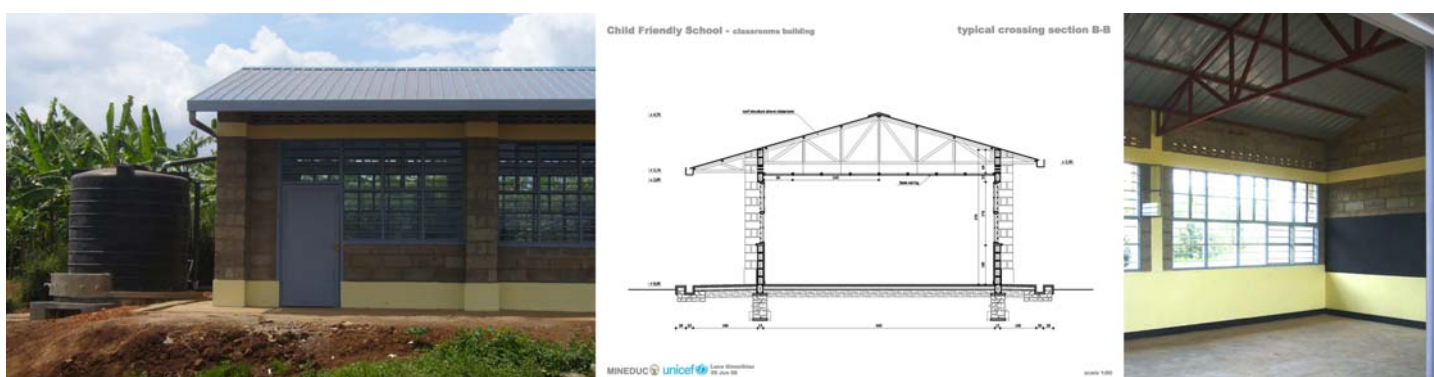
Typical UNICEF Child Friendly School roof metal structure with BG-28 metal sheeting and rain harvesting system
