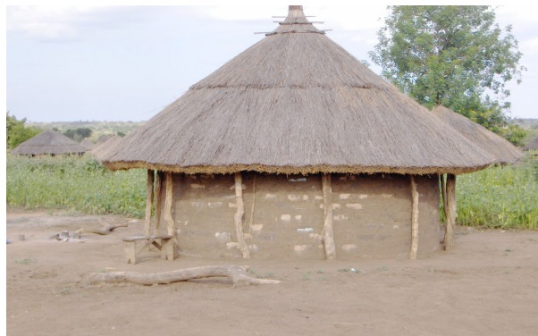
Figure 2 New house constructed for the elderly widow.
